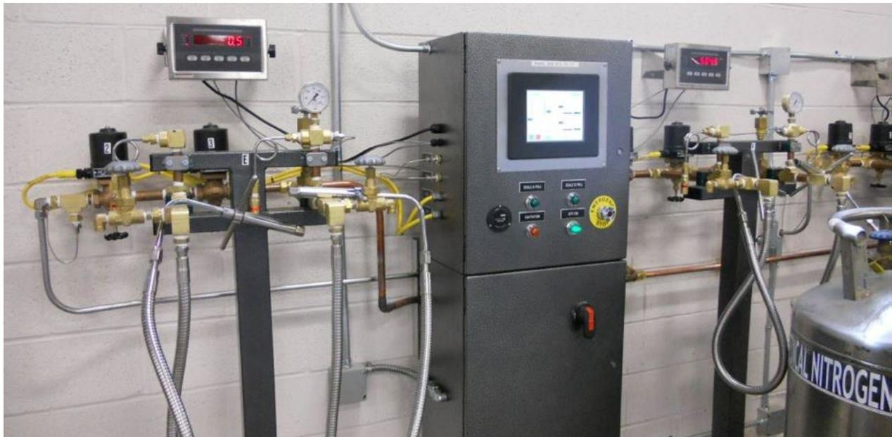
*Liquid cylinders that have a low working pressure (22-50 PSI) should be filled by the "bottom fill" method with the vent valve open to allow continual venting during fill.*
